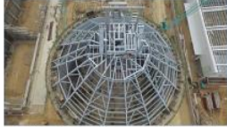
Clinker Silo Roof Project - Thilawa SEZ
