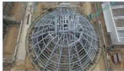
Clinker Silo Roof Project - Thilawa SEZ
