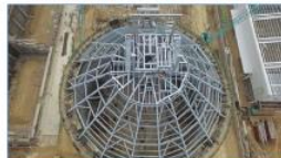
Clinker Silo Roof Project - Thilawa SEZ
