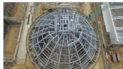
Clinker Silo Roof Project - Thilawa SEZ
