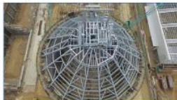
Clinker Silo Roof Project - Thilawa SEZ
