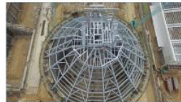
Clinker Silo Roof Project - Thilawa SEZ
