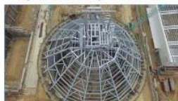
Clinker Silo Roof Project - Thilawa SEZ
