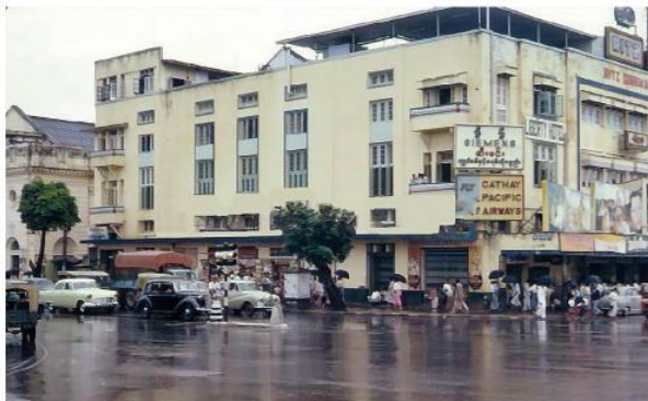
Before the construction of the Sakura Tower in the 1980s. Age-old cars make you feel its age
