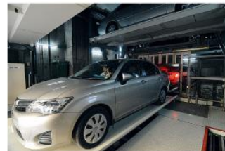
◀ Also equipped with a Japanese-made mechanical parking lot that can hold 78 cars. Because there are few parking lots in downtown, it is one of the grateful facilities.
