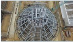
Clinker Silo Roof Project - Thilawa SEZ
